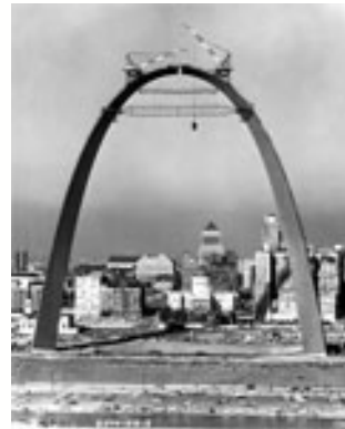
United States Jefferson National Expansion Memorial, St. Louis, Missouri, under construction, 1965 From the Collections of Arteaga Photos Ltd.
