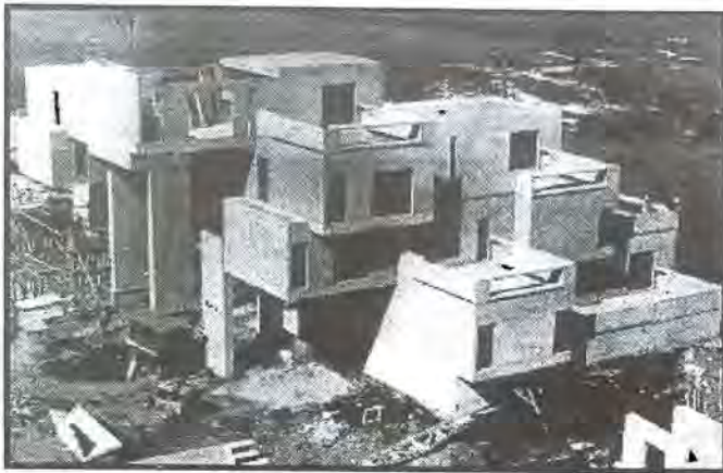
Construction of Habitat '67 at the Montreal Expo
