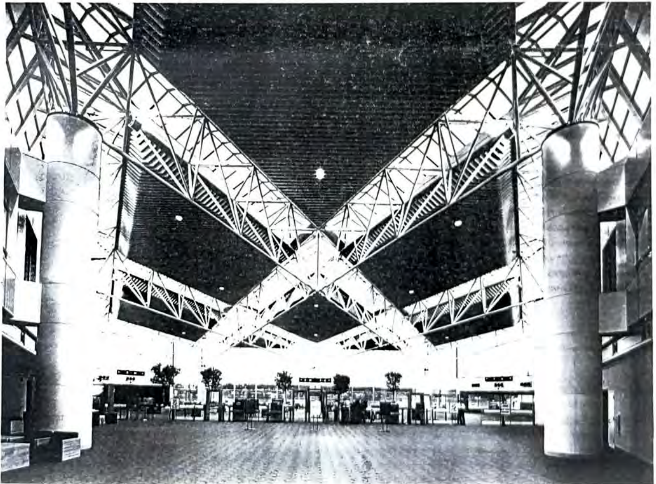
Concourse D, Interior
