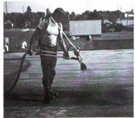
MONOFORM protecting "spirits" warehouse — Milwaukie, Oregon
